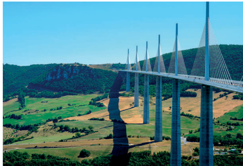
Life Cycle assessment of bridge decks: Advantages of PVA-FRC over conventional systems [2] (Possible application)
